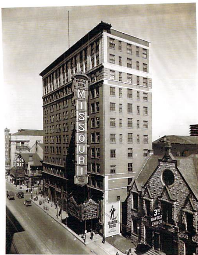
Exterior of the Missouri Theatre, 628 N. Grand Boulevard. The Grand Central Theater can be seen immediately to the north, with an advertisement for Show Boat. The St. Louis Theatre, now Powell Hall, is immediately north. Photograph by W. C. Persons, 1929. Missouri Historical Society Collections.
