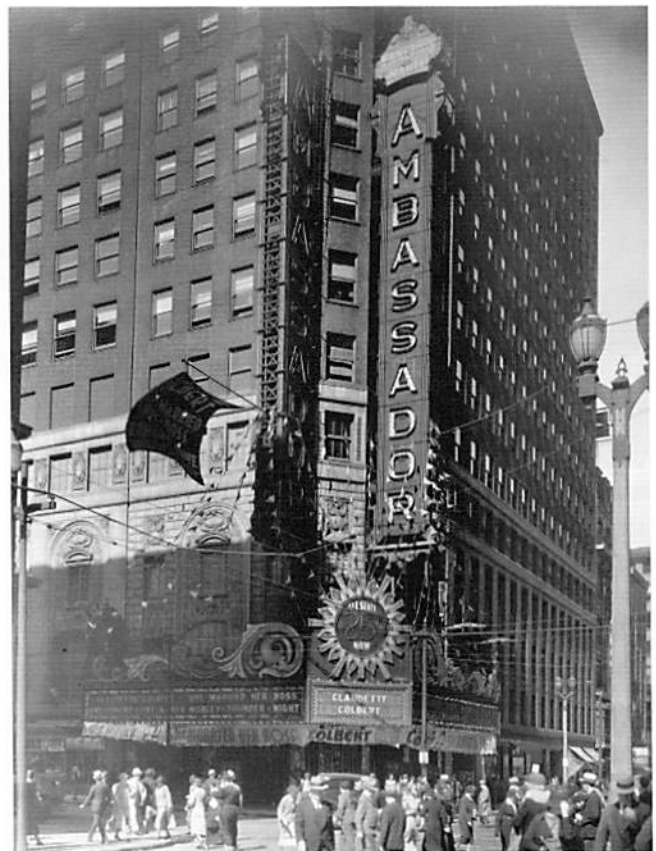
Exterior of the Ambassador Theater, at the northwest corner of Seventh and Locust streets. Photograph by W. C. Persons, 1935. Missouri Historical Society Collections.
